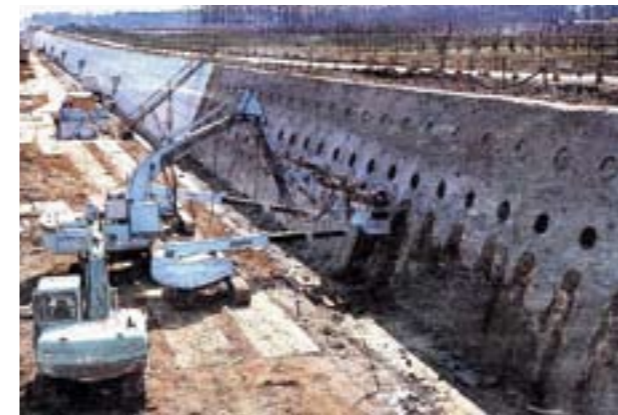
Nail-reinforced soil wall under construction (for Tohoku Line of high speed train) 既設のり面急勾配化工法の事例(東北新幹線)
