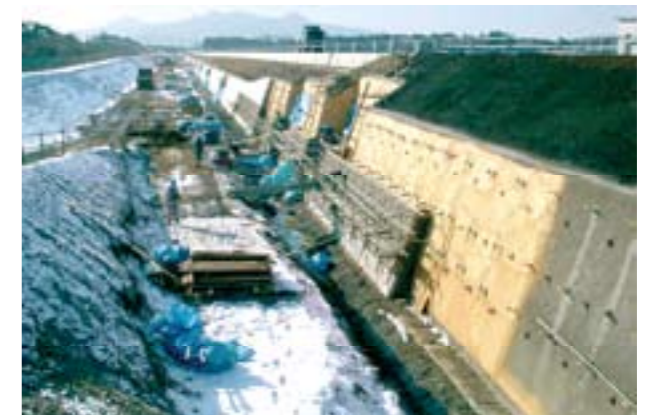
Nail-reinforced soil wall under construction (for Tohoku Line of high speed train) 既設のり面急勾配化工法の事例(東北新幹線)
