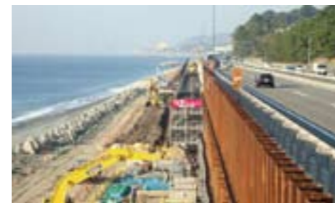
施工状況 During construction
