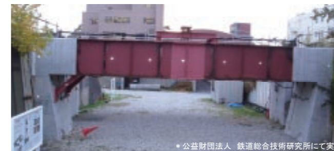
Full-scale model of Integral Bridge with Nail - Reinforced Soil (NRS Integrated bridge) 既設盛土一体化橋梁(NRS一体化橋梁)の実物大模型
